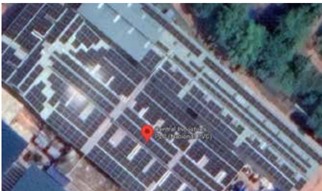
Solar energy system, Factory premises, Yakkala
