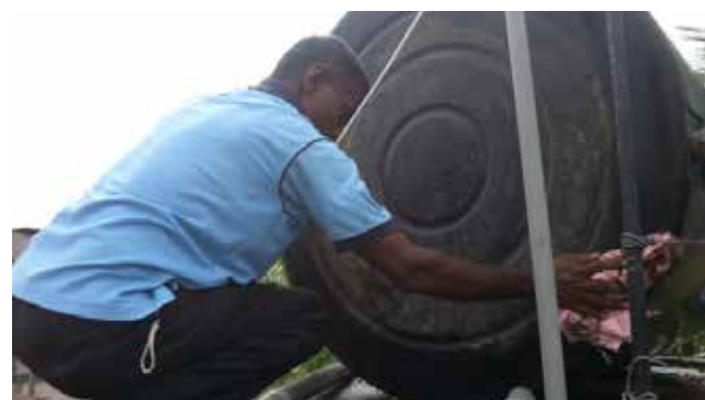
Repairing of a water tank (for extended usage even beyond the terms of the warranty)
